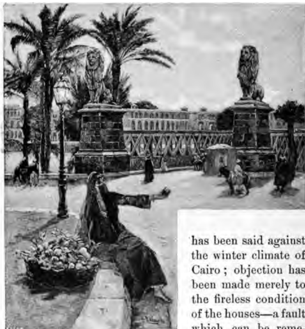
THE NILE BRIDGE, CAIRO From a photograph by Sebah, Cairo
